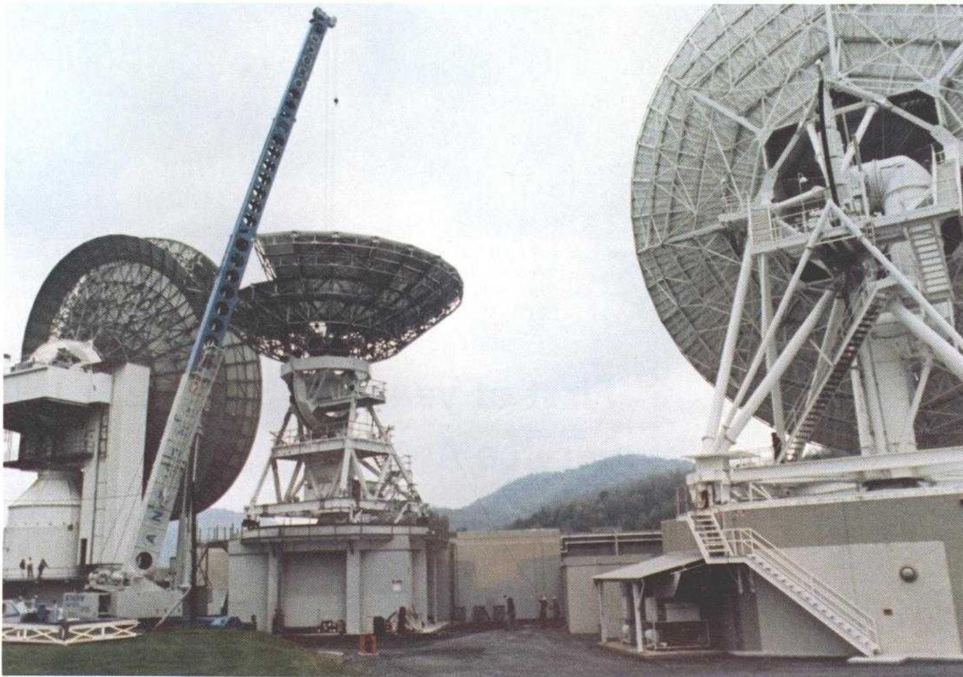
*Dish reaches its final position atop alidade and concrete pedestal. Flanking new Standard C antenna are Etam's two Standard A antennas.*
